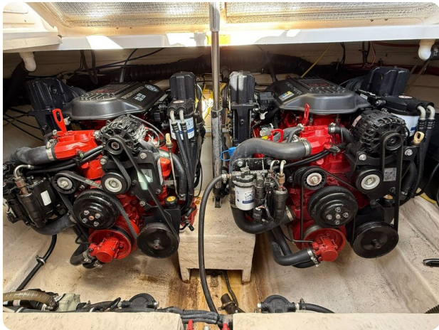
CHAPARRAL SIGNATURE 310 Engine room
